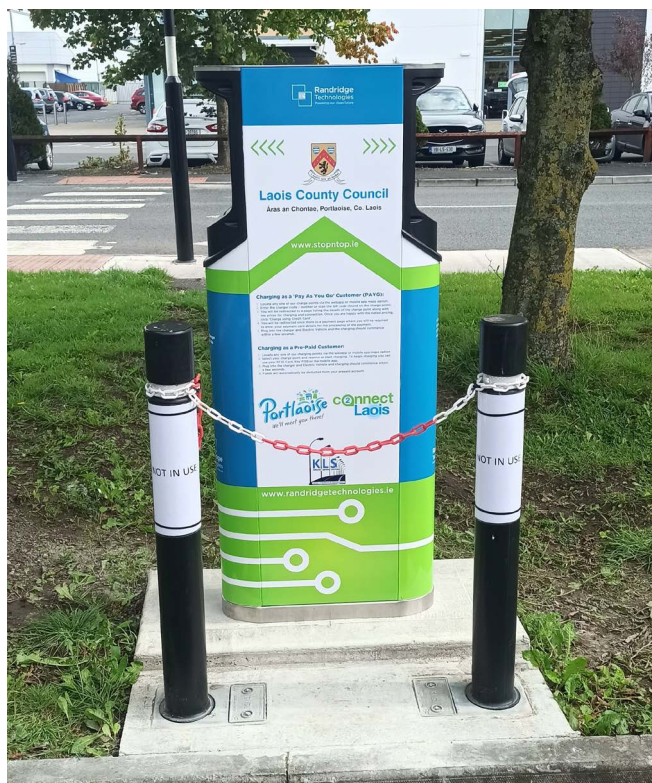
Figure 16: 2 x 22 kW on-street EVCP, Portlaoise - Laois CC (Source: Laois CC)
