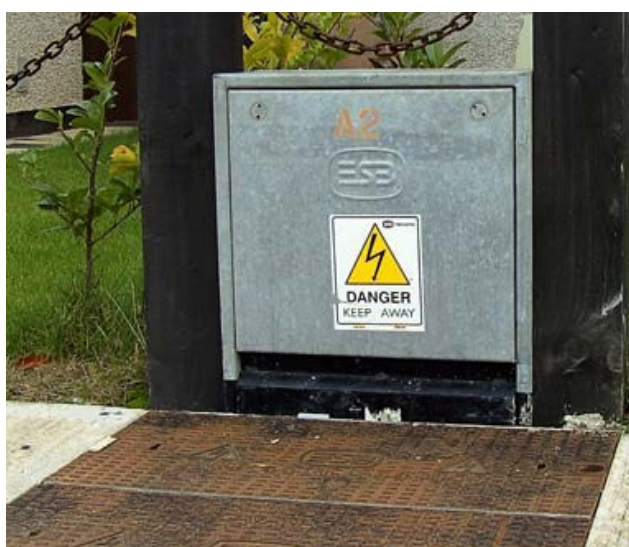
Fig 24: ESB Mini pillar (Source: ESB Networks)
