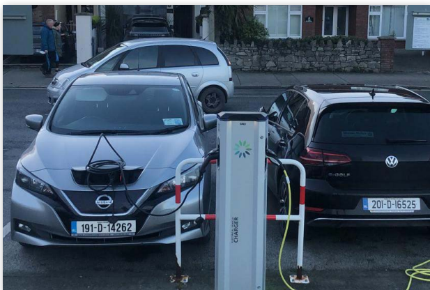
Figure 29: 2 x 7kW on street EVCP Skerries - (Source: Fingal CC)
