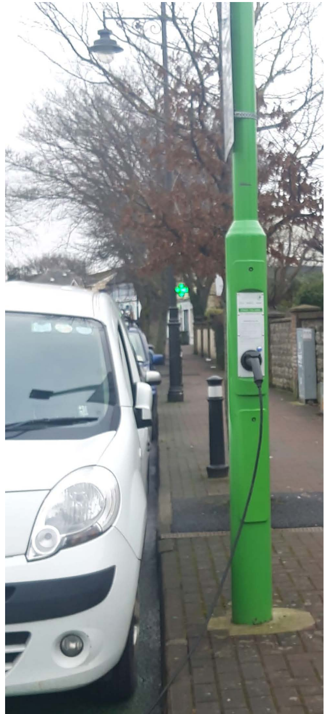
Figure 18: On Street Smart pole EVCP installed by Fingal CC at Blanchardstown, North Co. Dublin (Source: Fingal CC).
