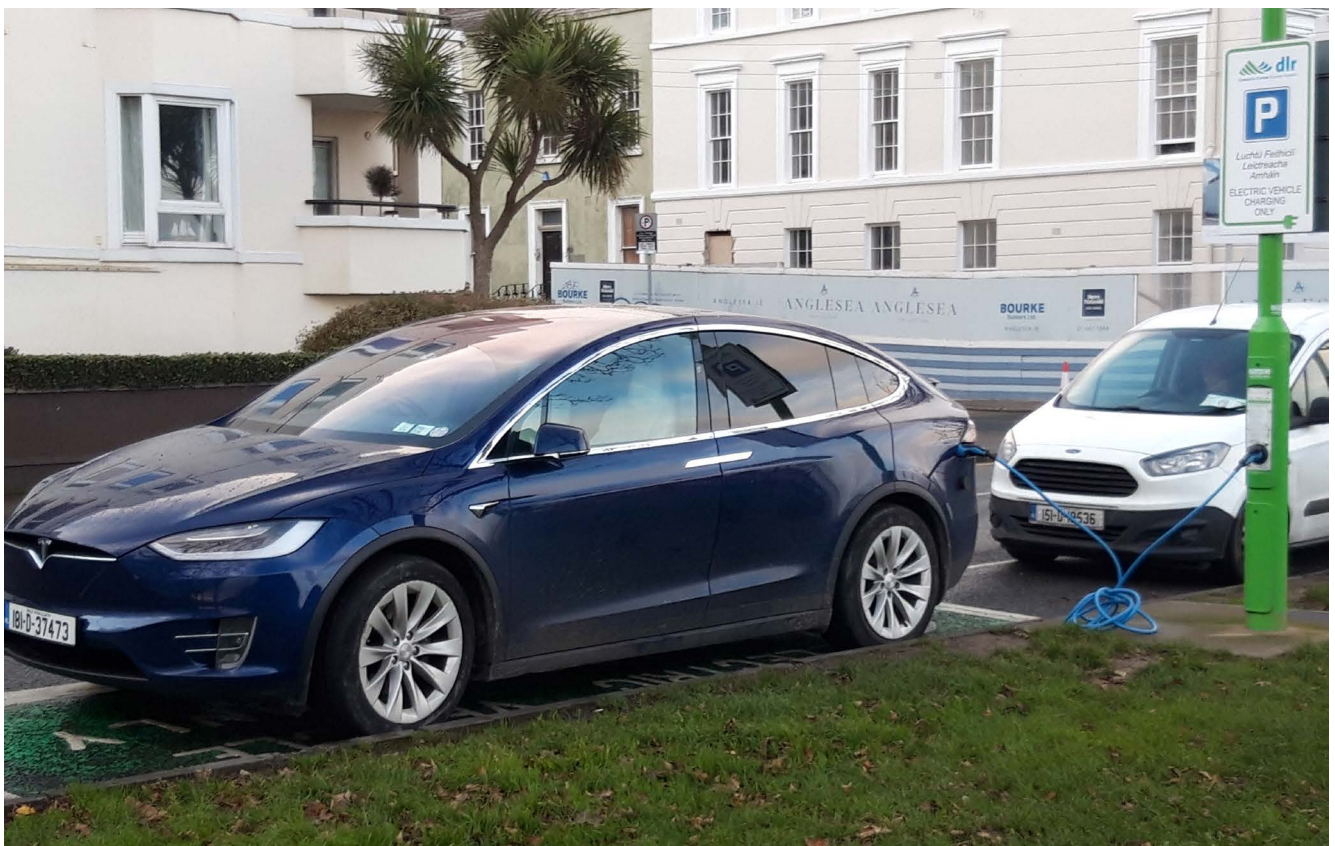
Figure 17: 7kW Smart Pole EVCP Dun Laoghaire – DLRCC (Source: Dublin CARO)
