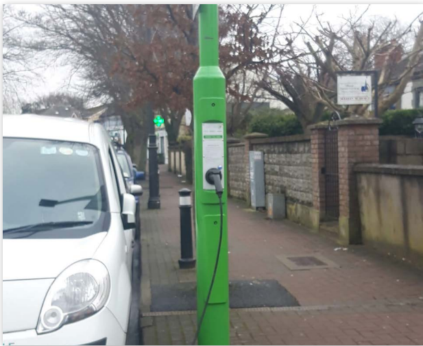
Figure 28: Smart Pole Charging Blanchardstown - (Source: Fingal CC)
