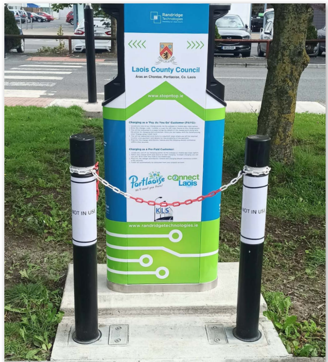
Figure 30: 2 x 22 kW on-street EVCP Portlaoise - Laois CC (Source: Laois CC)
