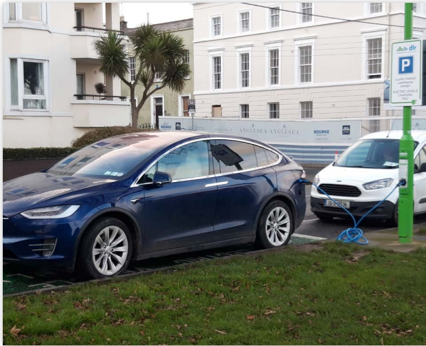
Figure 26: 7kW Smart Pole EVCP Dun Laoghaire – DLRCC (Source: Dublin CARO)
