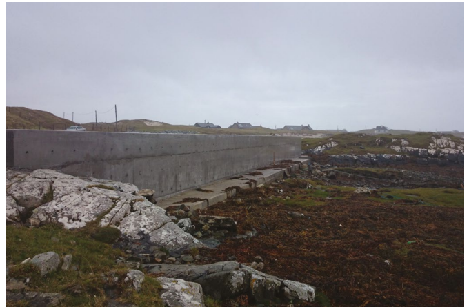
Figure 4 Examples of coastal engineering solutions (source: Arup): Beach nourishment works with shingle in Greystones beach (upper left); and breakwaters Greystones Harbour Co. Wicklow (upper right); T shaped Groyne in Penrhyn (UK) (bottom left), concrete wave wall Aillebrack Co. Galway (bottom right).
