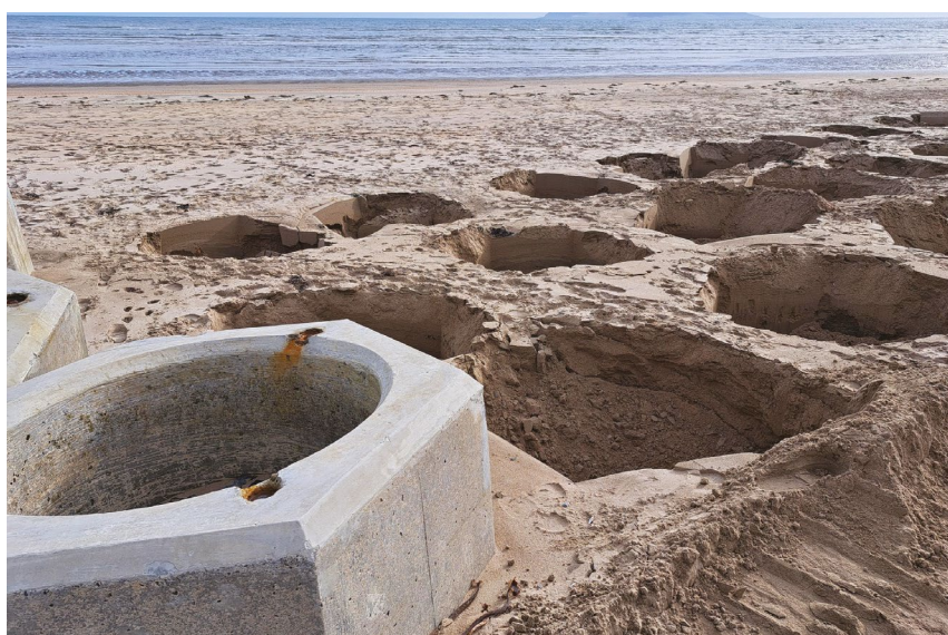
Figure 7 Seabee Units, East Coast of Ireland
