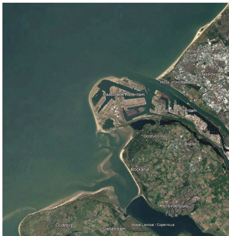
Figure 25 (Right) GE image of the Maasvlakte-2 Rotterdam Port extension
