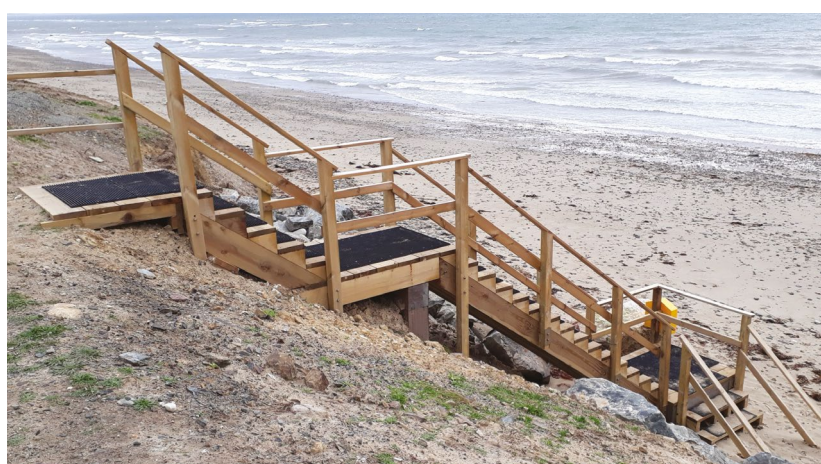
Figure 13 Seaview Temporary Access steps in 2018
