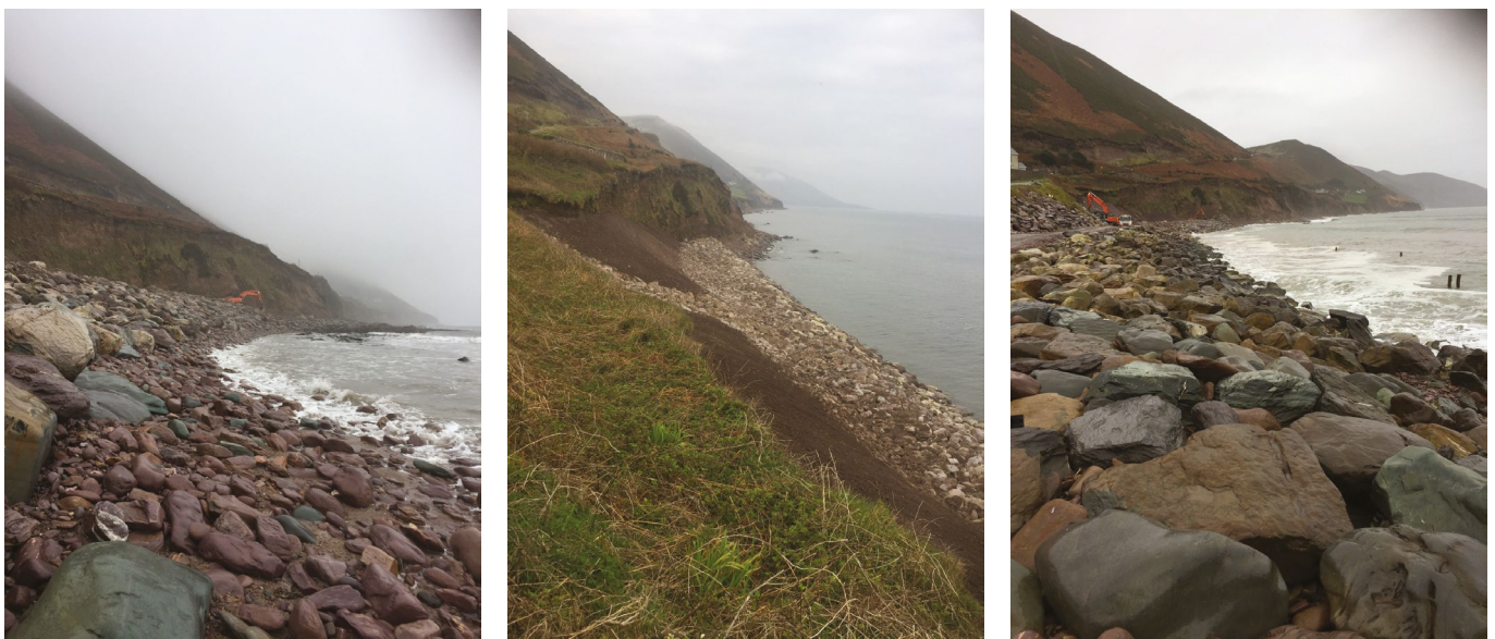
Figure 10 Coastal Protection Works at Rossbeigh
