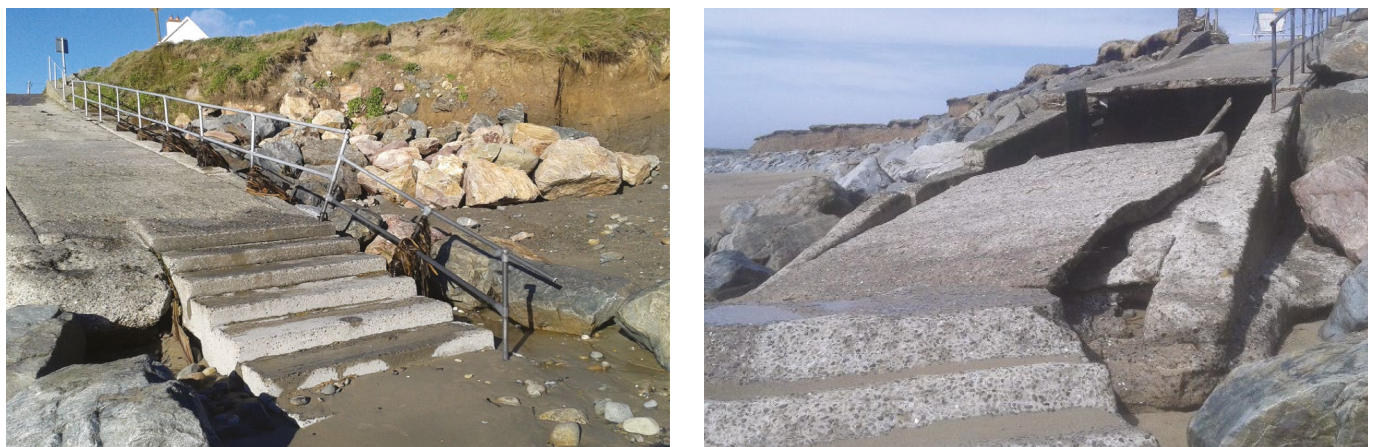
Figure 12 Beach access steps 2013 (left) and 2018 (right)
