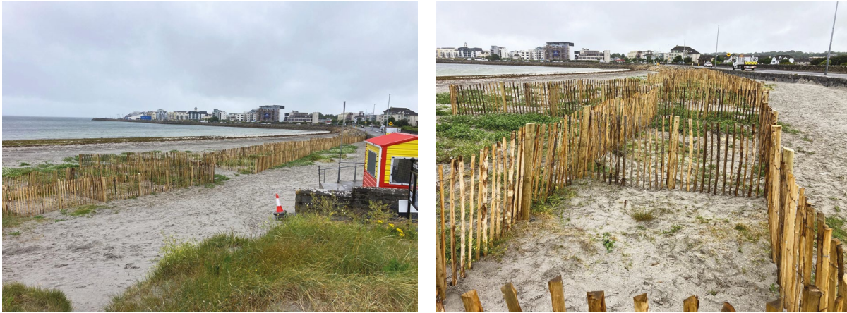
Figure 20 Light fences installed at Grattan Beach
