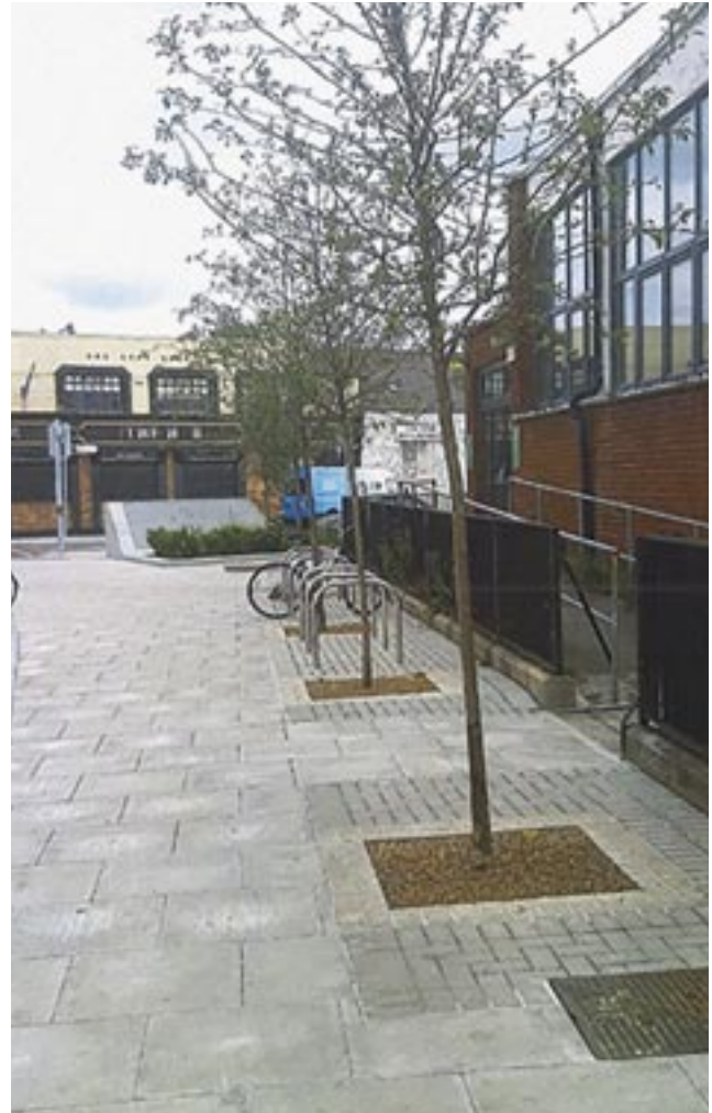
Figure 5.33: Tree pits for draining surface water.
