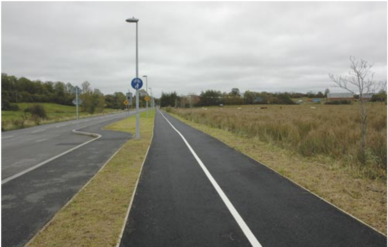
Figure 5.22: Segregated cycling lanes, Carrick-on-Shannon.
