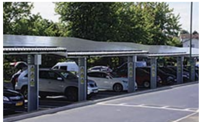
Figure 5.15: Flexisolar car park installation example.
