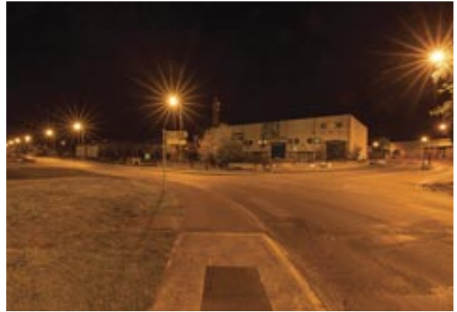
Figure 5.9: Hebron Industrial Estate, Co. Kilkenny – non-LED lighting.
