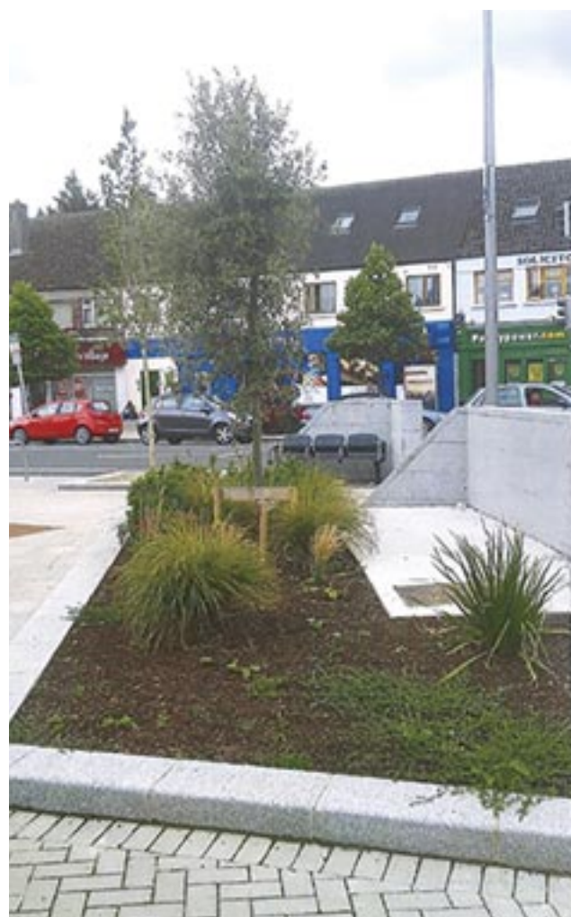
Figure 5.32: Green engineered flood defences – Crumlin Village.
