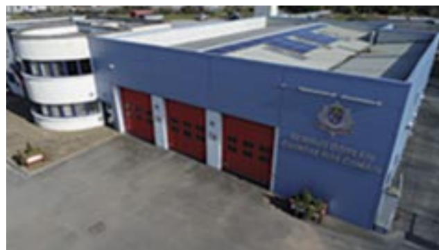
Figure 5.12: Aerial view of solar PV panels, Roscommon Town Fire Station.
