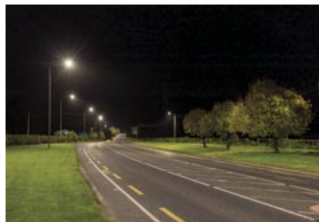
Figure 5.6: Clara, Co. Kilkenny – LED lighting.
