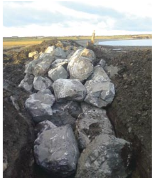
Figure 5.30: Construction of rock armour wall – Kilcredaun, Co. Clare.
