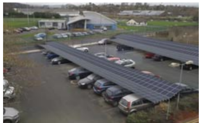
Figure 5.16: Proposed view, car park PV panels.
