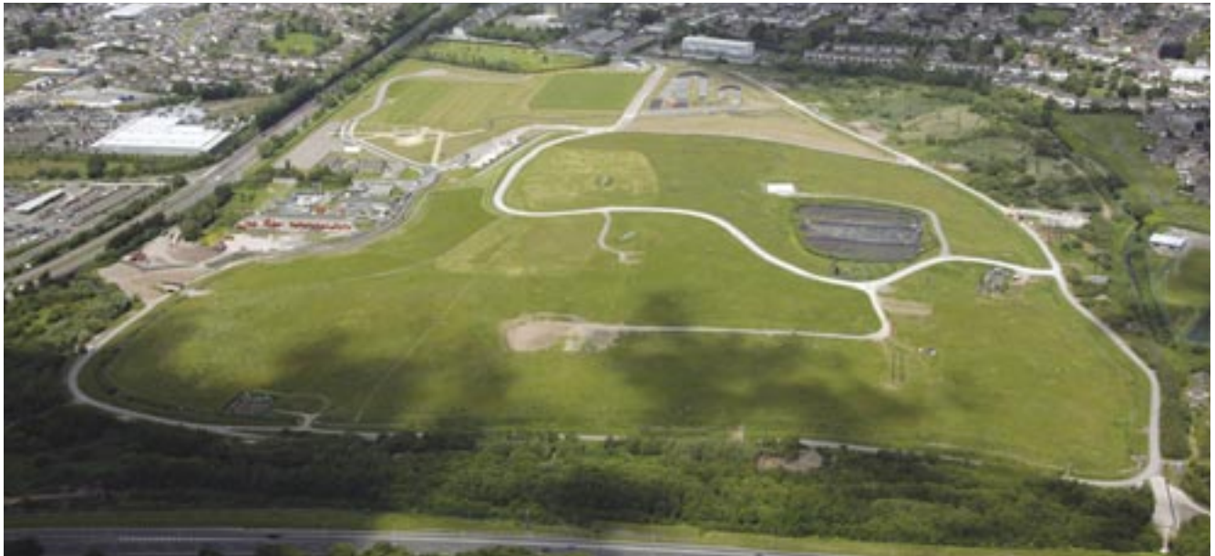
Figure 5.44: Aerial view – Tramore Valley Park, Cork City.
