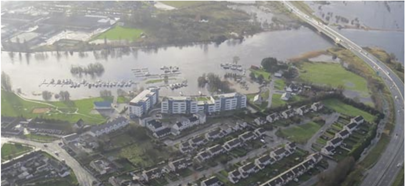
Figure 5.35: Flooding – Athlone, Co. Westmeath.
