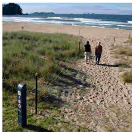
A fence design that has minimum impact on the environment and is easy and low cost to erect and maintain may be all that is required in even high use areas. This low cost fence comprises waratahs placed 10 m or more apart with two conspicuous yellow cords, is easy to maintain and move as the dune vegetation expands or the dune erodes. In addition, accessway signs encourage pedestrians to keep to formalised routes to and from the beach.
