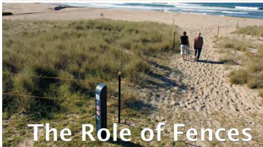
A fence design that has minimum impact on the environment and is easy and low cost to erect and maintain may be all that is required in even high use areas. This low cost fence comprises waratahs placed 10 m or more apart with two conspicuous yellow cords, is easy to maintain and move as the dune vegetation expands or the dune erodes. In addition, accessway signs encourage pedestrians to keep to formalised routes to and from the beach.
