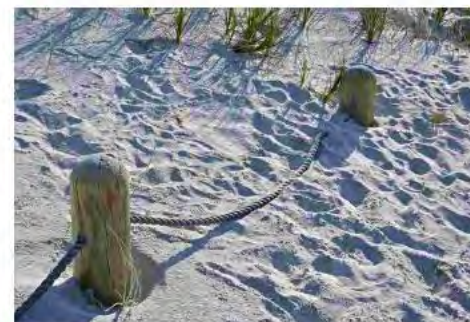
Regular inspection and maintenance of all fence types is essential so that they continue to protect dune vegetation from pedestrian and vehicular traffic effectively. Where sand is accumulating, bollards and posts will require lifting. Broken rails will require replacement and broken wires or cord restraining.
