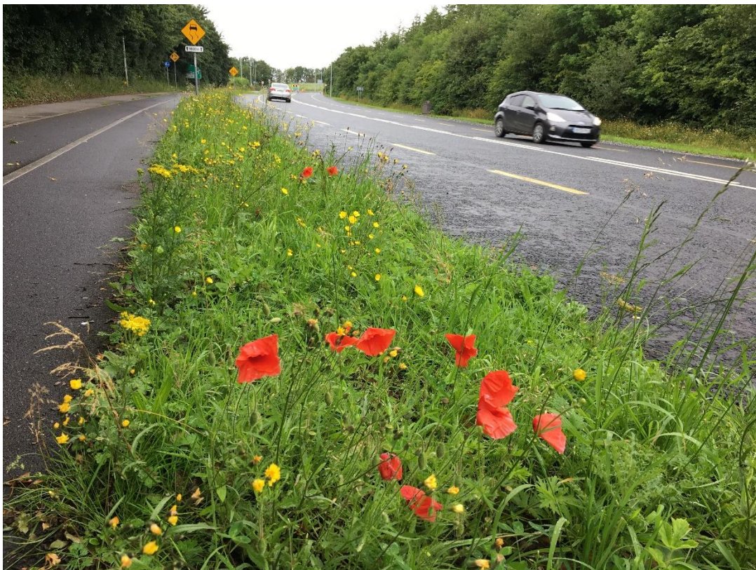
Vegetated filter strip on N24, Clonmel, Tipperary also provides biodiversity and aesthetic benefits. Integrating NBS can bring multiple benefits if a multidisciplinary approach is taken.
