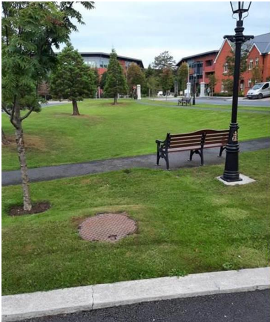
A well-established and well-maintained detention basin adds amenity (The Way, Citywest Avenue, Citywest, Dublin 24)
