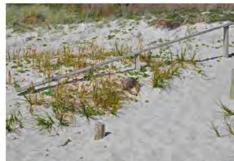
Regular inspection and maintenance of all fence types is essential so that they continue to protect dune vegetation from pedestrian and vehicular traffic effectively. Where sand is accumulating, bollards and posts will require lifting. Broken rails will require replacement and broken wires or cord restraining.
