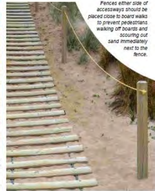
A fence design that has minimum impact on the environment and is easy and low cost to erect and maintain may be all that is required in even high use areas. This low cost fence comprises waratahs placed 10 m or more apart with two conspicuous yellow cords, is easy to maintain and move as the dune vegetation expands or the dune erodes. In addition, accessway signs encourage pedestrians to keep to formalised routes to and from the beach.
