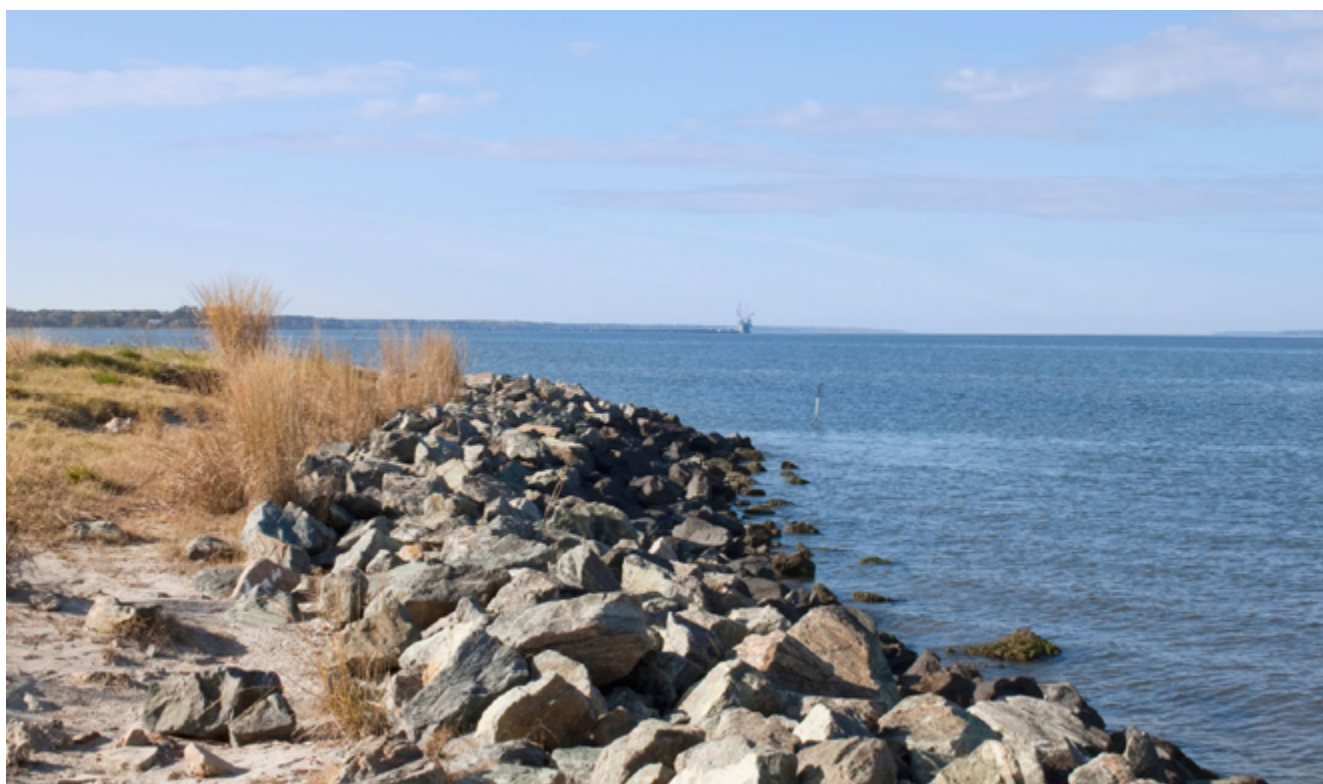
Image: Rock wall for protection from erosion and tidal surges in Chesapeake Bay, Maryland
