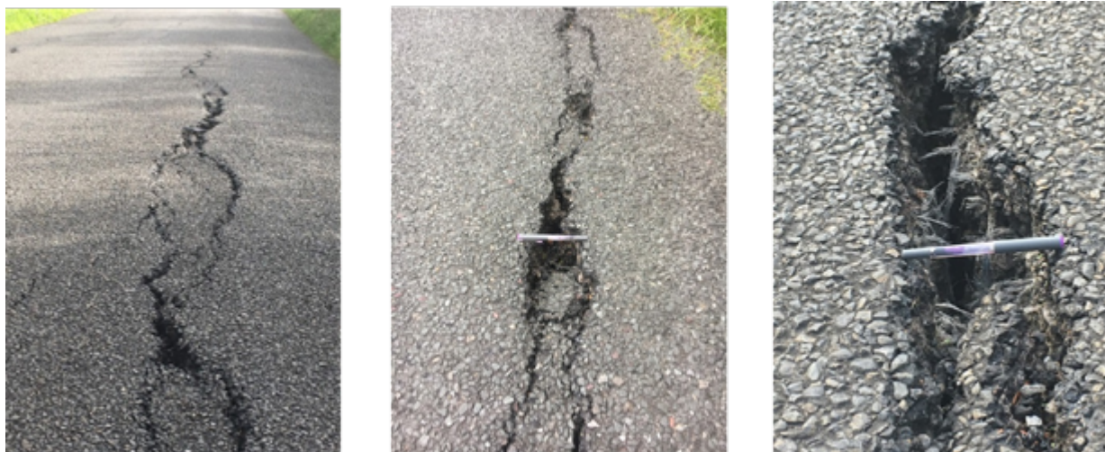
Image 1: Horizontal Cracking from extreme and prolonged heat on road over bogland 2018 (Offaly).
