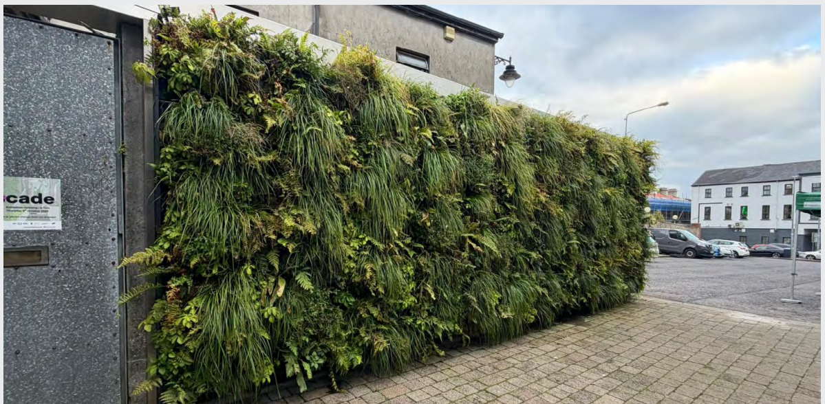
Photo: Green wall NbS part of Cascade urban rainwater project Ballina, Co. Mayo
