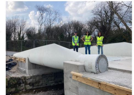
Walking on wind blades. Re-Wind Network's first BladeBridge pedestrian bridge was installed in Cork, Ireland in Jan. 2022. Photo Credit: Re-Wind Network.
