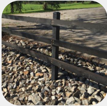
Fencing posts with painted timber runners
