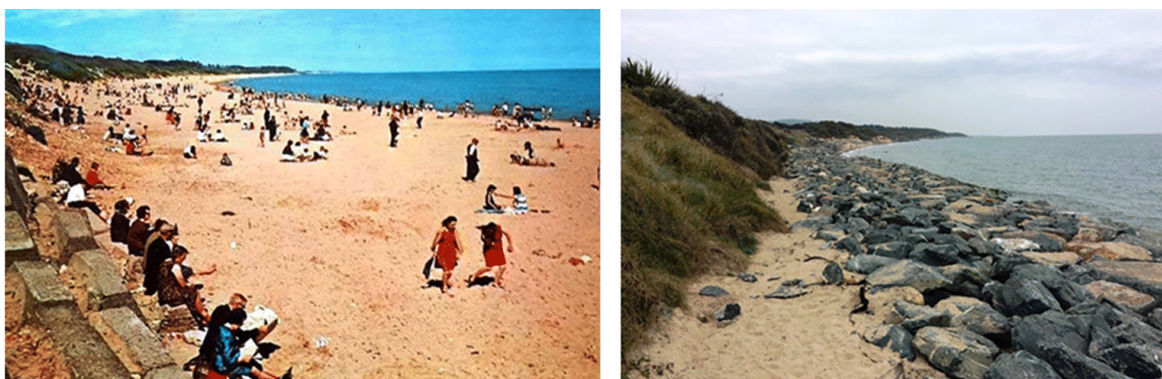
Figure 6 North beach at Courtown in 1967 (left) and in 2015 (right) with rock armour. Source: Phillips and Murphy (2021)
